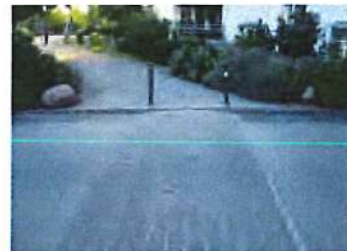
Speed tables work to both slow down traffic as well as provide a clear pathway way for pedestrian travel. They can be adopted for both residential and urban conditions.
