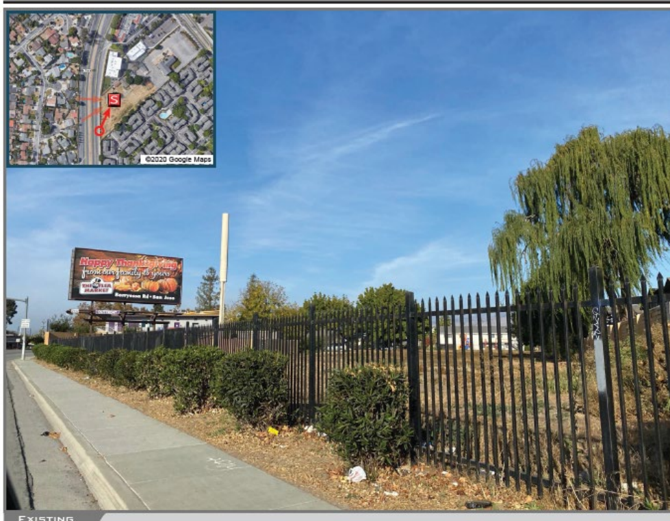
Figure 1 – The existing monopole and radome.
