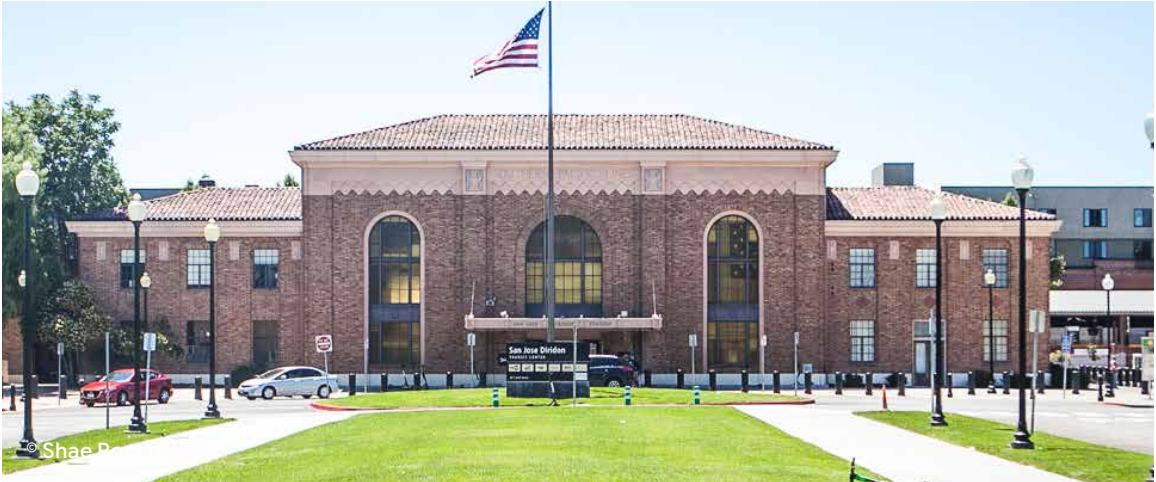
D. SOUTHERN PACIFIC STATION (65 CAHILL STREET)
