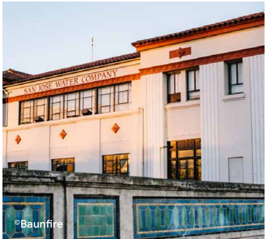
C. 374 WEST SANTA CLARA STREET (WATER COMPANY BUILDING)
