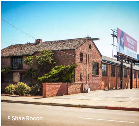
A. 150 SOUTH MONTGOMERY STREET (HELLWIG IRONWORKS)
