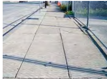
Existing Conditions, Montgomery Street Source: Fehr & Peers, 2010
