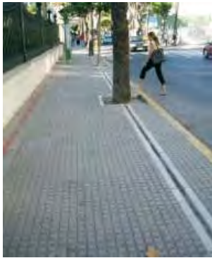
Consider the integration of rain water collection systems such as bioswales and rills into the streetscape.
