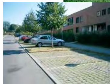
The use of pervious materials in surface parking areas increase water infiltration and decrease the heat island effect. Different pavement for street parking also visually narrows the street.
