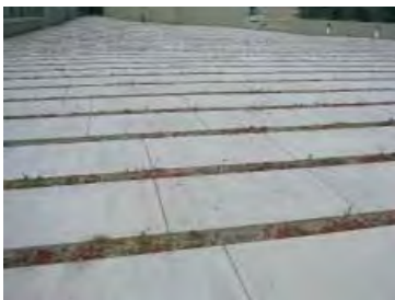
Permeable paving can help to reduce urban runoff while creating a distinctive look.
