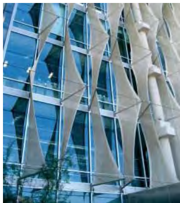
Shading devices that are integrated in the façade significantly reduce energy consumption.
