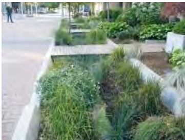
Bioswales retain rain water and reduce the impact on the storm water system. If designed well, they can improve and green the streetscape.
