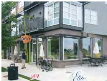
Ground floor retail should have no setbacks to the street and wrap around the building corner.
