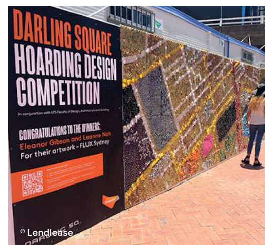
TEMPORARY CONSTRUCTION SIGNAGE
