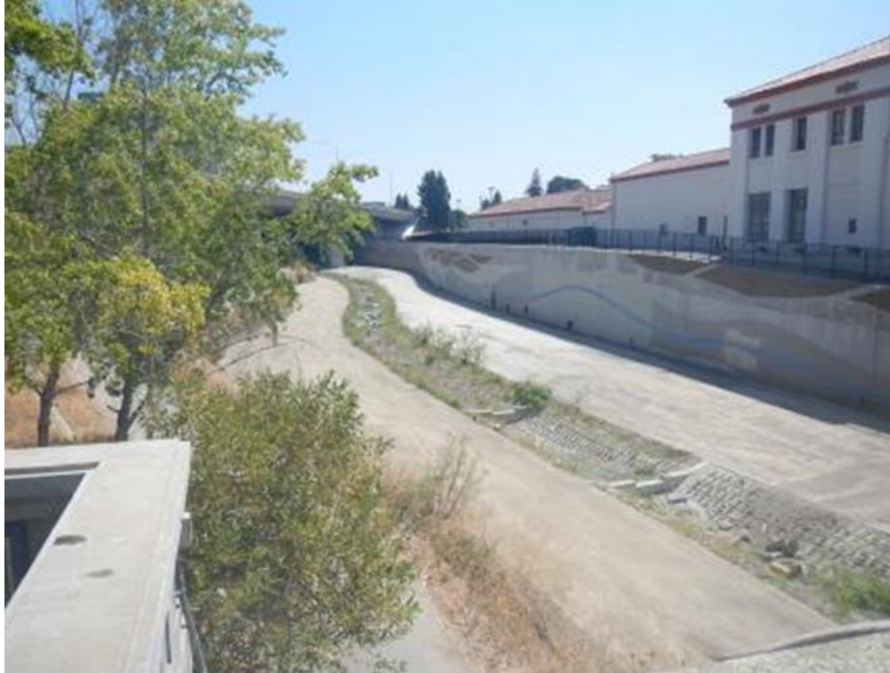
1. Guadalupe River, looking south. Concrete floodwall and existing buildings at Project site west of river. Portion of Guadalupe River Trail and landscaped riverbank east of river.
