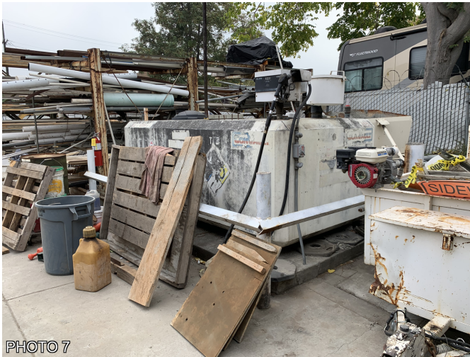
FUEL ABOVEGROUND STORAGE TANK
