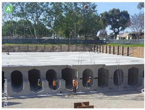
Example of Subsurface Infiltration Chamber under Large Green Space at Bolivar Park in Lakewood, California
