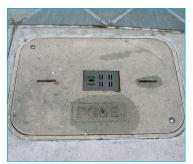
PG&E Gas Meter. Concrete Enclosure and Lid
