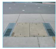
PG&E Subsurface Transformer. Incential traffic Lid – Polymer/Concrete Finish
