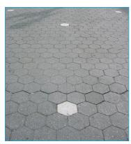
Hexagonal asphalt paving is the standard for paving Paseos (or approved equivalent)
