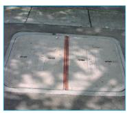
B48D2. 2pc. Reinforced Concrete (Cable) Concrete Enclosure and Lids
