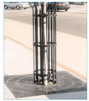
The approved San Jose tree grate, Boulevard Collection Model R8713 with the approved Model "C" tree guard both from Neenah Foundry
