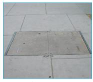
PG&E Subsurface Vault Polymer/Concrete Finish
