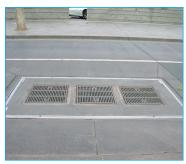
4'-6" x 8'-6" PG&E Transformer Cover Heavy Full Traffic. Code No.:04-1442 Polymer/Concrete Finish
